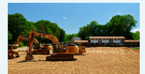
GH breaks ground on the Harrison Village.
